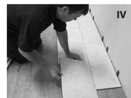
they are approximately 1/4" (6mm) apart. Click the tile lengthwise into place. For the short and long edge, use the tapping block and a number of smaller taps until the tiles lock into place completely.
