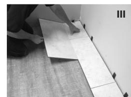
The cut piece from the first row may need to be cut to become the starting piece for another row. Install the cut edge facing the wall, with the expansion wedge in place. Now angle this piece and click it into the first tile of the first row (III). Continue the second row with a full piece, placing the tongue of the long side into the groove of first row piece (IV). Move the end joints together until
