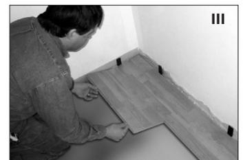
The cut piece from the first row becomes the starting piece for another row. Install the cut edge facing the wall, with the expansion wedge in place. Now angle this piece and click it into the first plank
