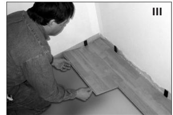
Click the plank lengthwise into place. For the short edge, use the tapping block and a number of smaller taps until the planks click into place completely.
