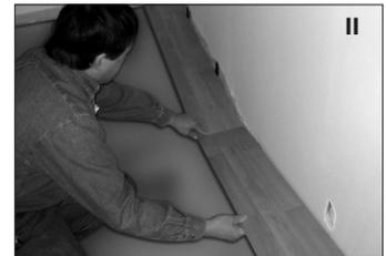
The cut piece from the first row becomes the starting piece for another row. Install the cut edge facing the wall, with the expansion wedge in place. Now angle this piece and click it into the first plank of the first row. The cut pieces should be a minimum of 8” (20cm) in length (III). Continue the second row with a full piece, placing the tongue of the long side into the groove of first row piece (IV). Move the end joints together until they are approximately 1/4” (6mm) apart.
